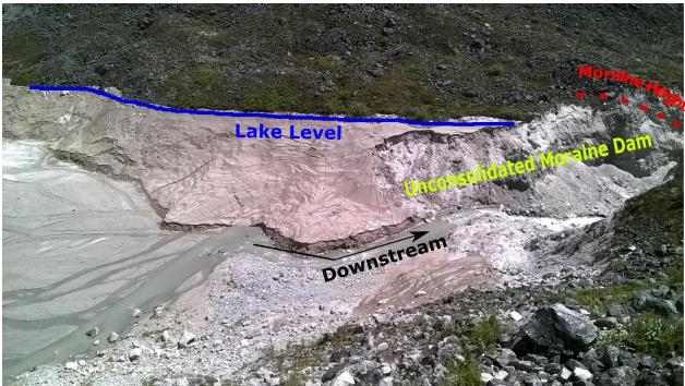
*Figure 3.2: Remnants of Lemthang Lake after the GLOF. Blue line shows the original Lake level and the dotted red line shows the original moraine dam height near the outlet.*
